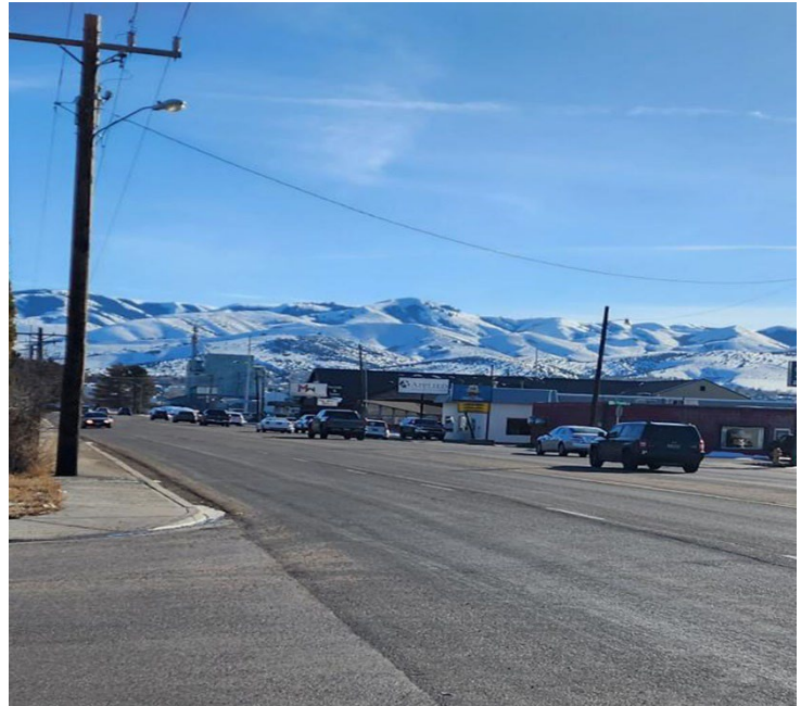
Figure 17 Low Power Lines over Pole Line Road
